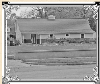
Renovations in process, 2017.
